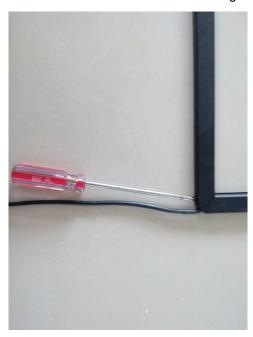
4.Next is the top left corner. Put the aluminum angle under the connecting wire. Fix the wire with the clip. Then fasten the screws.
